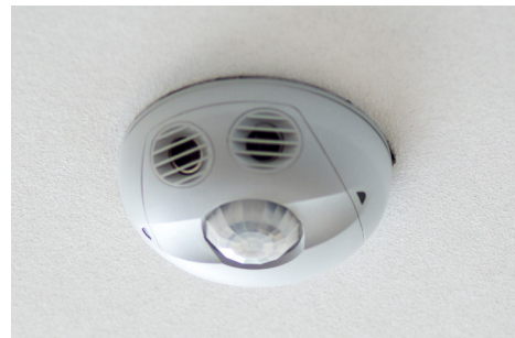
A lighting vacancy sensor saves energy by automatically turning off lights when a room is empty.
