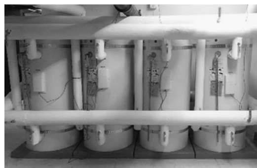
Indoor hot water storage tanks.
