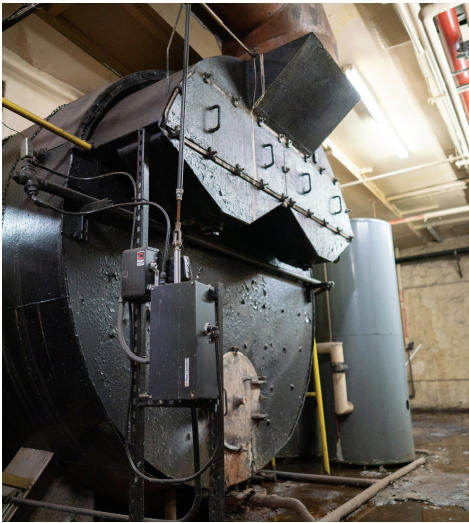
Replacing an aging boiler will enhance efficiency.
