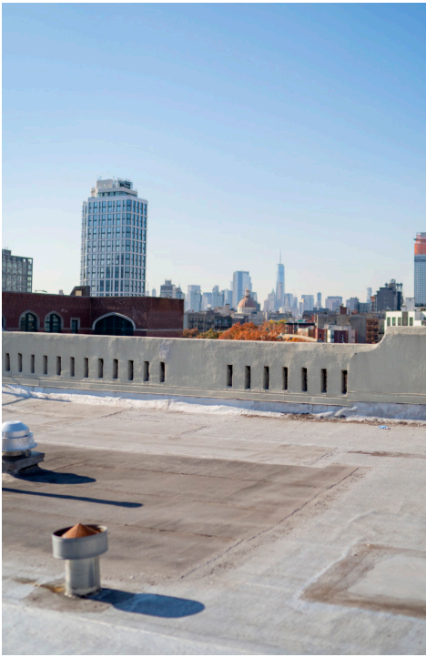
Plans to upgrade the building roofs with enhanced insulation and greater reflectivity will help maintain consistent indoor temperatures and prevent heat transfer.
