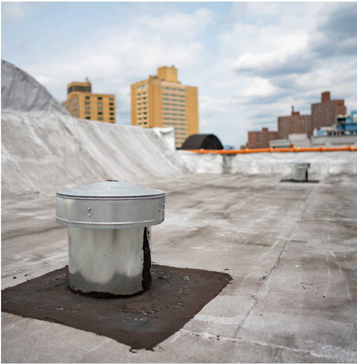
Improved roof insulation helps increase occupant comfort and reduce energy costs.
