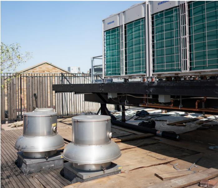
Air-source heat pumps improve energy efficiency and reduce carbon emissions.
