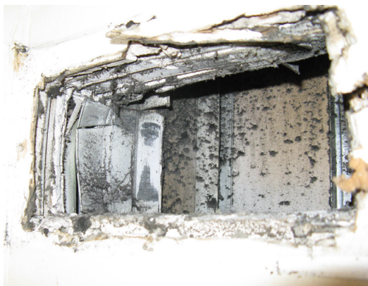
View into a dusty, grimy air duct.
